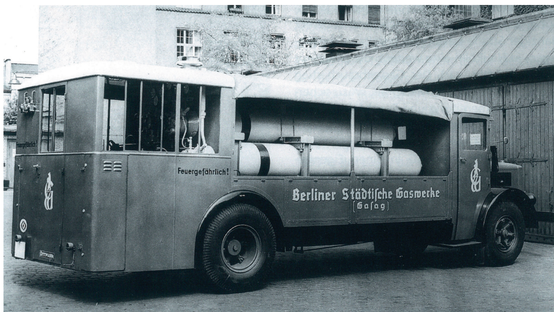
Figure 3: A gas-powered lorry of the Berlin gas utility used to deliver gas to filling stations. Source: Hilmar Bärthel, Die Geschichte der Gasversorgung in Berlin. Eine Chronik (GASAG Berliner Gaswerke Aktiengesellschaft, Berlin: Nicolai, 1997), 93.
