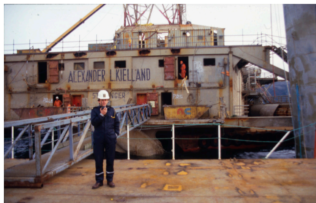
Figure 4: Inspection of the rig after it was turned right-side up. Photo: Sven Tønnessen / Norwegian Petroleum Museum (NOMF-02641.27_1).
