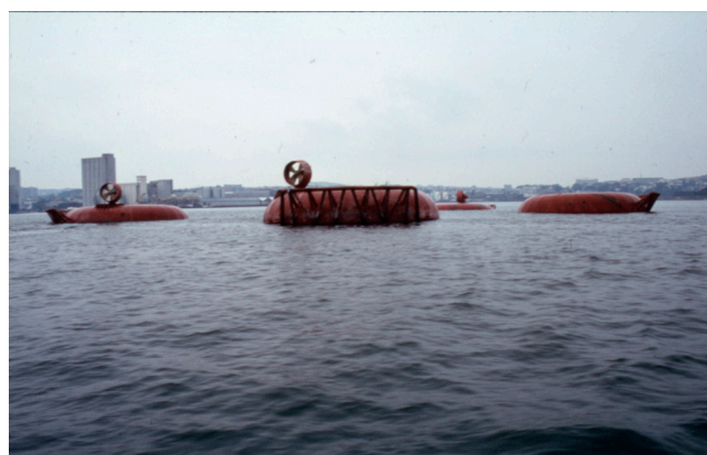
Figure 3: After the capsizing. The rig was towed ashore upside down. Only the buoyancy elements on the columns were visible. Stavanger Drilling II AS & Co owned this rig as a limited partnership with several stakeholders. The 'Alexander L. Kielland' rig was stationed on the Ekofisk field operated by Phillips Petroleum Company. Photo: Sven Tønnessen / Norwegian Petroleum Museum (NOMF-02641.02_04).
