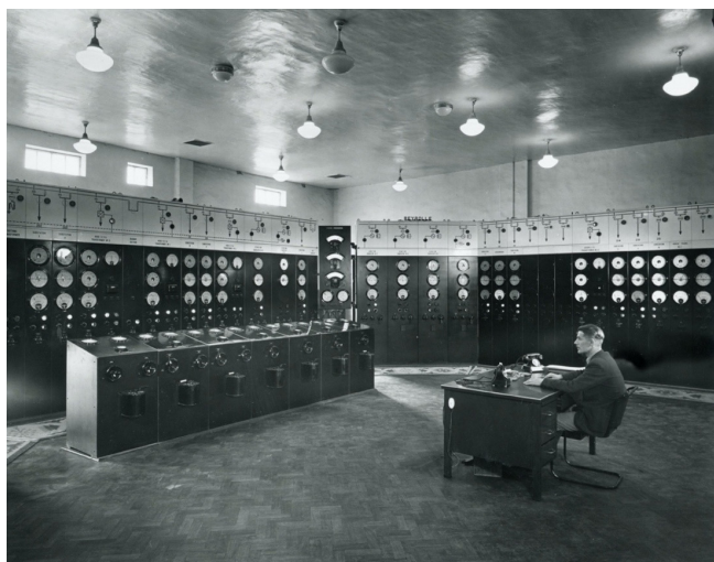
Figure 3: Automation in Abadan: inside the refinery power station control room, late 1940s. Source: BP 115890B.
